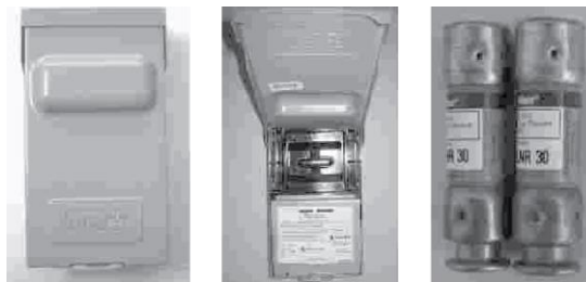
Disconnect switch box for outdoor unit
