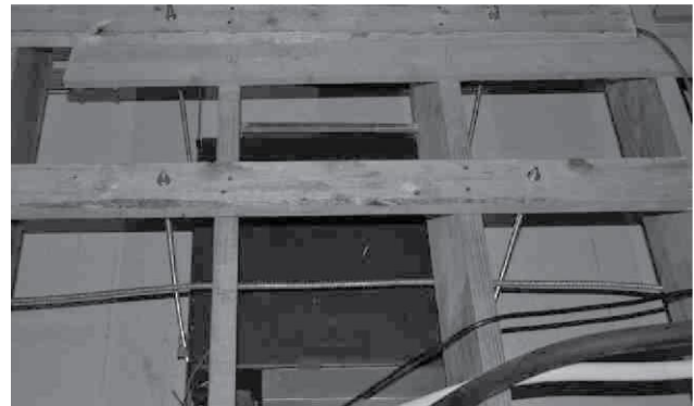
Mounting-Threaded Rod Hung on Rafters
